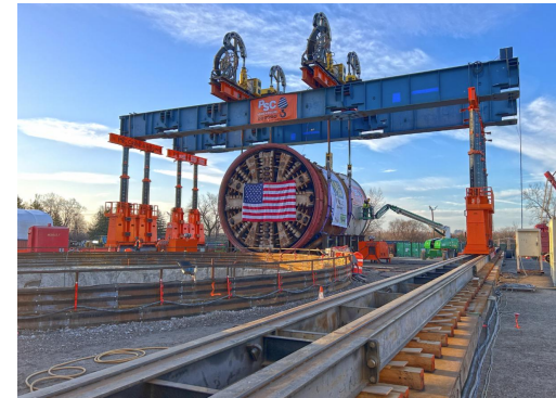
Cleveland TBM preparing to be lowered.
