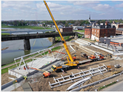
City of Piqua Lock No.9 Project from April of 2024.
